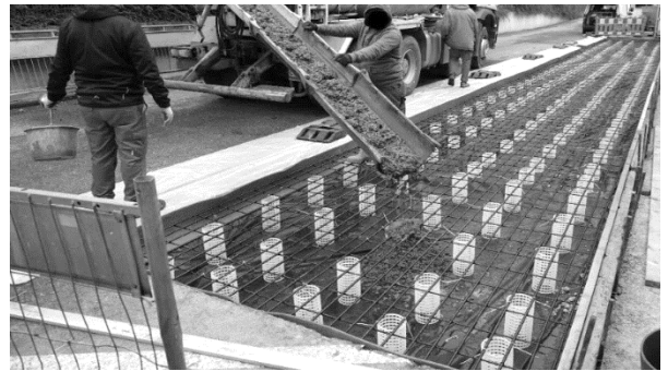
Figure 14: Plastic filter tubes as supports for a metal-free component
