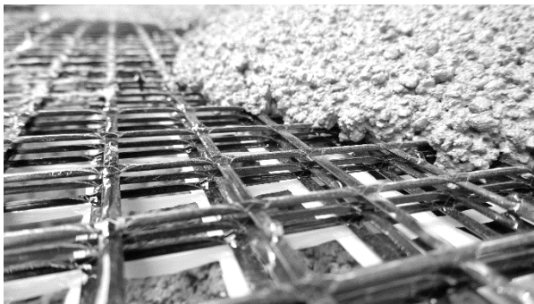
Figure 20: Plane support of reinforcement grids using grids as spacers
