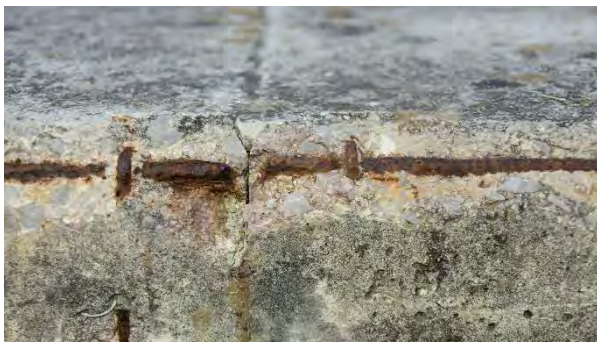
Figure 2: Consequences of reinforcement corrosion
