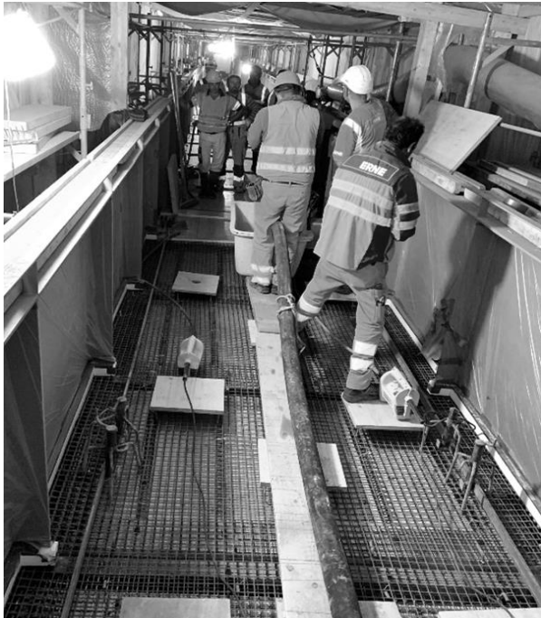
Figure 19: Access aids to prevent direct access to reinforcement made of fiber-reinforced composites
